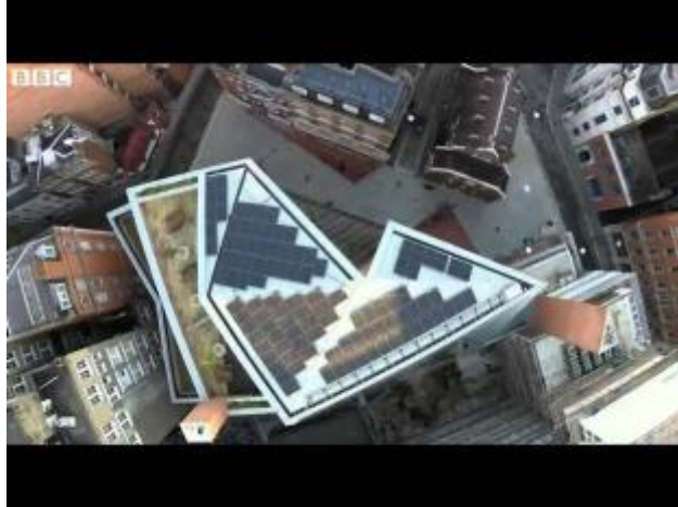
1 - Building the Everyman Theatre
